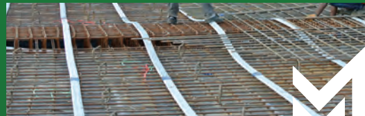
SLAB & SPIRAL DUCT
